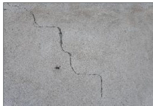
Non-structural Crack
