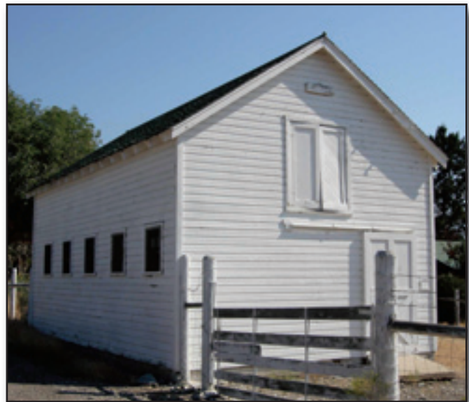
Figure 1—Following national trends, the Forest Service often used wood siding with a variety of profiles on frame buildings in the early 20th century. The drop siding on this barn was one of the most popular choices. The barn was built in 1933 at the Salmon Ranger Station in Salmon, ID (Salmon-Challis National Forest, Intermountain Region).
