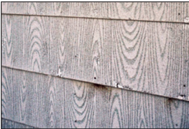
Figure 7—The wood-grain pattern on these asbestos siding shingles makes them look similar to wood shingles when viewed from a distance.
