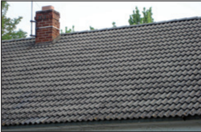
Figure 6—Asbestos-cement roofing tiles were popular on period revival styles such as the Mission and Spanish Eclectic styles, which were most common in the Southwest and Florida.
