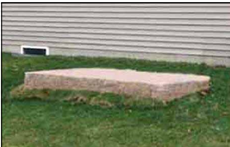
Figure 3-4. Concrete Pad Site
