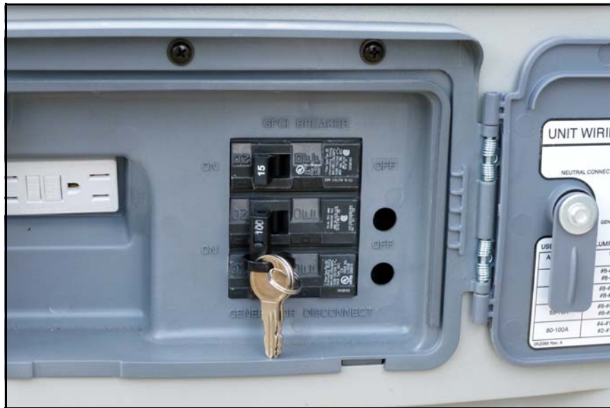
Figure 2-3. Circuit Breaker Box and Keys (As Shipped)
