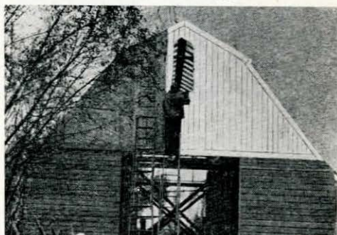
Fig. 36. The right way —This farm owner is painting as soon as siding is on his new corn crib. A priming coat applied to the siding before it is nailed on saves much labor. With only a small outlay for equipment, regular farm help can be utilized on the painting job.
