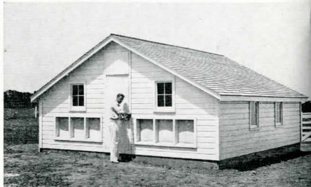
Fig. 17. Typical Farm Security Administration poultry house, properly painted. Not only is good paint economical from the standpoint of service, but it is a labor-saver when the time comes to repaint. It provides a firm, solid base that need not be scaled off before the new coat is applied.
