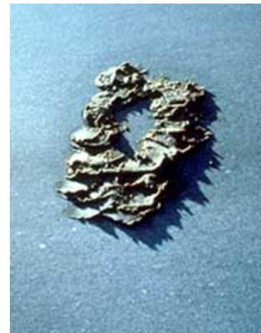
A poultice is often the preferred method of graffiti removal. Photo: NPS files.
