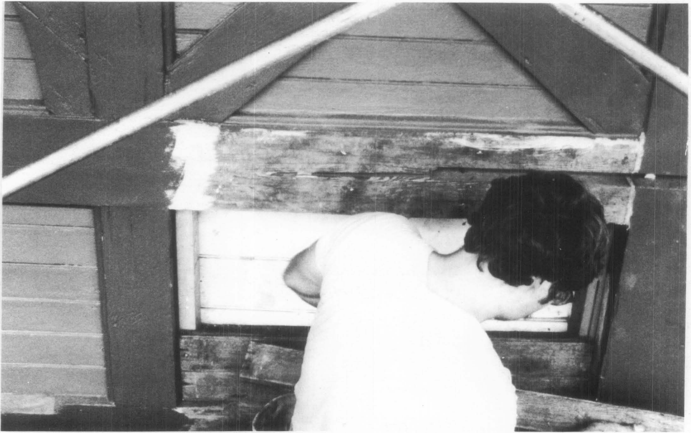
Figure 6. Sound pieces of wood salvaged from elsewhere on the building are being used to replace this deteriorated tongue and groove panel. In most cases, deteriorated wood trim, sills, and paneling were replaced with redwood that was back primed. Photo: Bryan Blundell
