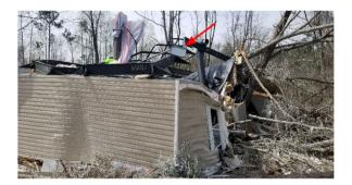
Fig. 2. Example pan system on manufactured/mobile home that experienced catastrophic failure (Overturning).
