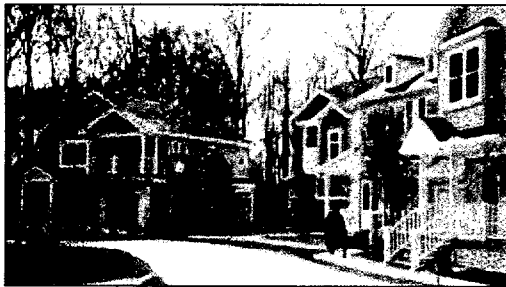
Two-story HUD-Code homes, Howard County, Maryland, 1997
