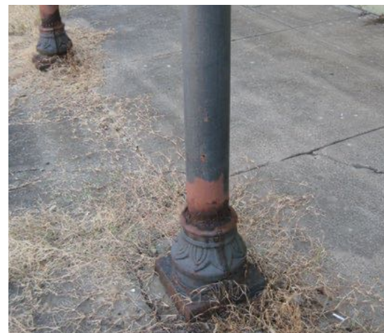
[7] (a) After the damaged portions of the base were repaired, (b) the cast-iron columns were cleaned and repainted to protect the metal from rusting.
