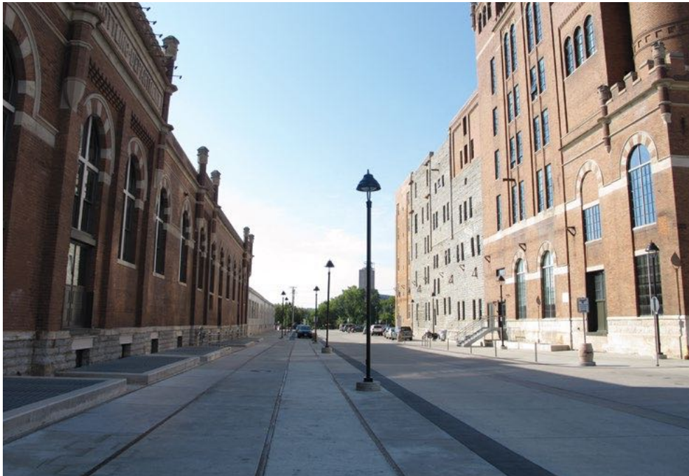
[43] The industrial character of the site was retained when this brewery complex was rehabilitated for residential use.
