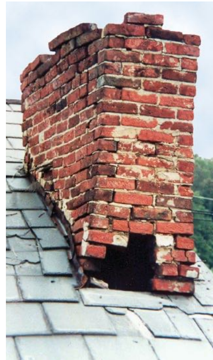
[7 a-b] This crumbling chimney was restored to its historic appearance using matching bricks.
