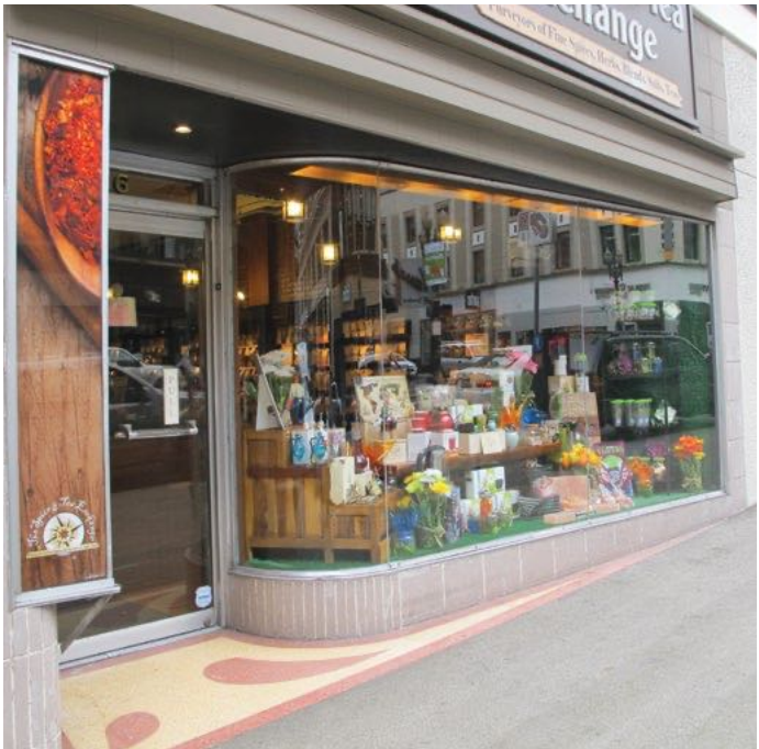
[27] This original c. 1940s storefront, with its character-defining angled and curved glass display window and recessed entrance with a decorative terrazzo paving, is in good condition and should be retained in a rehabilitation project.
