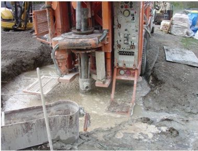
Figure 12-6 shows the back of an orange coloured drilling rig. A black coloured drilled well casing extends out of the muddy water through a rotary table. The drilling rig is holding on to the casing with the rotary table and a welded piece of steel. During drilling the flow around the outside of the casing created a void in the ground. The overburden above the void has collapsed creating a 10 metre (30 foot) deep by 4 metre (13 foot) wide hole filled with water. The void was unknown until the time of overburden collapse. The void created a serious safety issue for anyone working on the back of the drilling rig.
