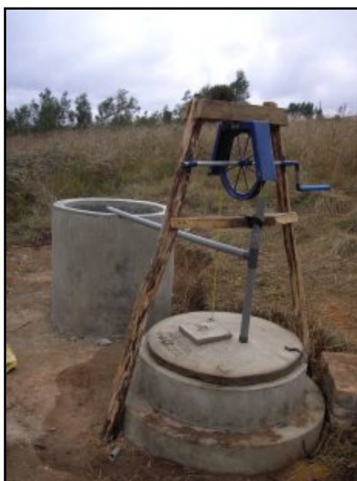
A hand dug well with Rope pump
