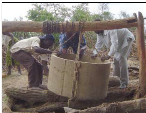
Lowering a well ring with a windlass
