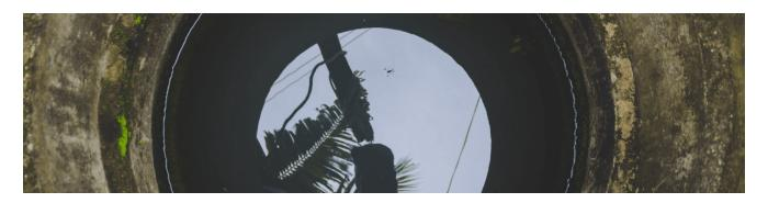
The water flow of potable and industrial underground water wells typically decreases over time. One of the main reasons for the decline in water productivity is the accumulation of scale, biofilm, clay, and iron oxide deposits. The contaminants block the water flow causing gradual damage to the water-well foundation and waterproducing formation.
