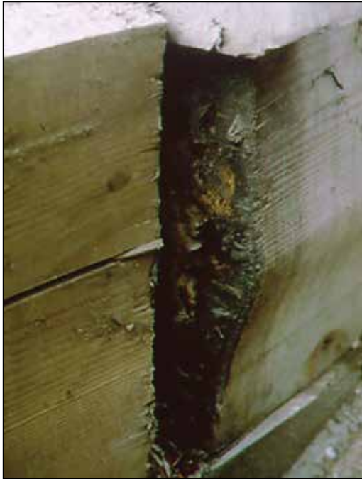
Figure 1.4—The timber beam's outer shell buckled as a result of interior deterioration.
