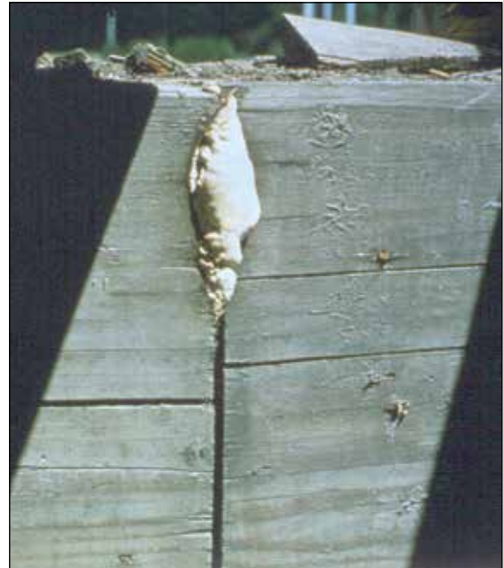
Figure 1.1—Fruiting body between two beams.
