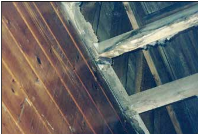
Figure 1.9—As a consequence of the moisture exposure, wood members in the roof and walls also contained areas of deterioration.
