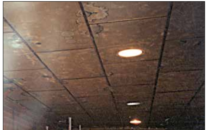
Figure 1.6—The ceiling panels were stained and discolored.
