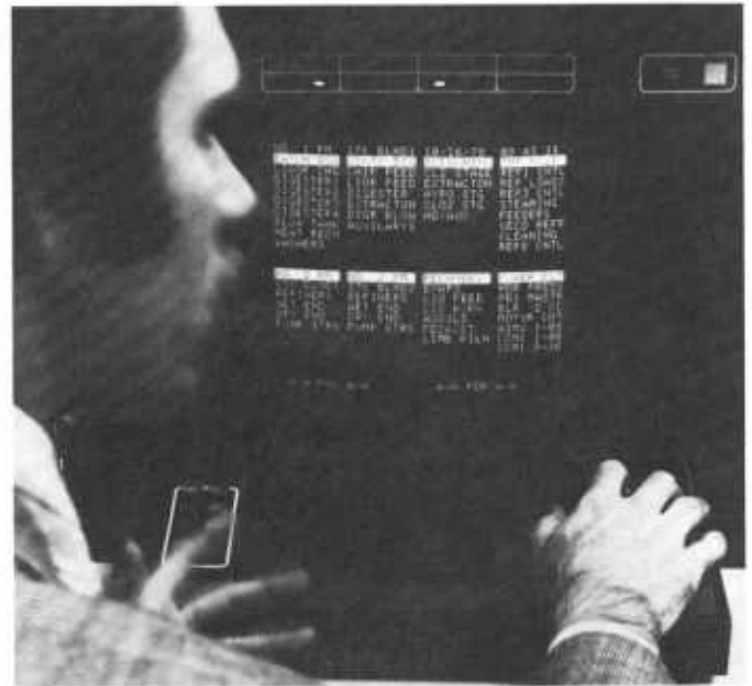
Figure 118—Plant area overview on video screen (Foxboro).
