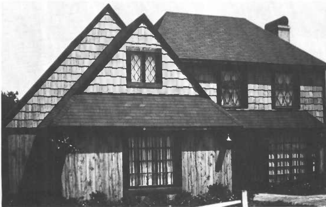
Figure 353 —Example of hardboard siding installation (Abitibi-Price Corp.).
