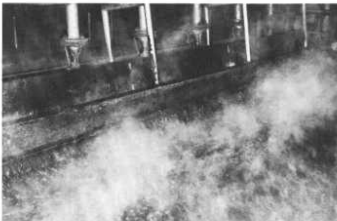
Figure 146 — Slush overlay being applied to S1S mat.
