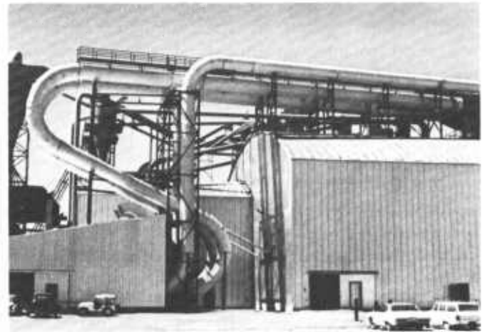
Figure 194 — Suspension tube flash-dryer in medium-density fiberboard plant (M-E-C Co.).
