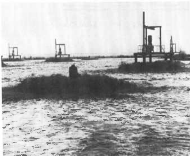
Figure 318 —Aeration lagoon with mechanical aerators.
