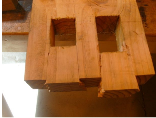
Figure 3-7: Full Tenon Relish Failure at each Keyhole
