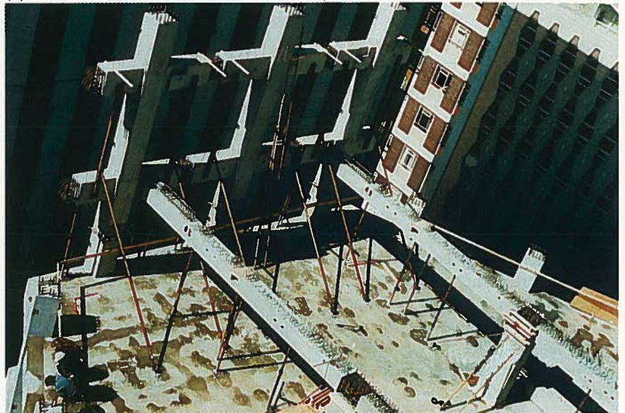
Fig. 9. Construction of a 13-story building using System 3 in New Zealand.
