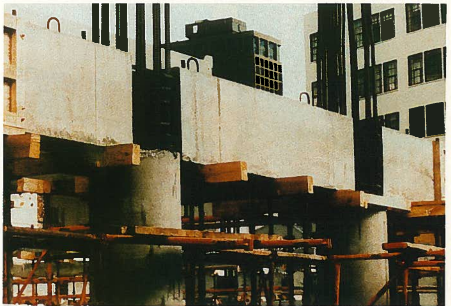
Fig. 5. Reinforced concrete building frame incorporating precast concrete elements in the beams between columns as used in System 1.
