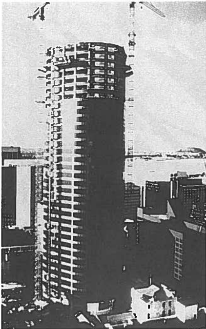
(a) Construction overview of building
