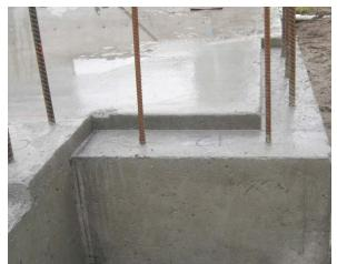
1.4 Panels are manufactured with cast-in Drossbach tubes (typically 3 x diameter of the starter bars) at nominated centres. These tubes fit over the starter bars, which are cast into the slab and extend 600 mm above the slab.
