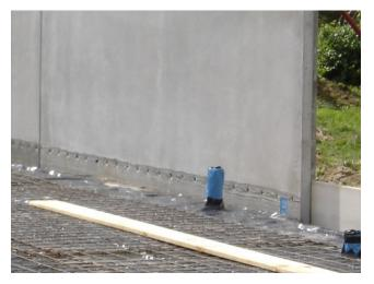
wall panels, working progressively around the foundation perimeter. See detail D(3)3 Panel/Floor Slab Connection. Props should not obstruct the pouring of the floor slab.
