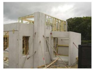
then the panels will require propping from the exterior face and attached to "dead men" positioned in the ground outside of the floor area, as shown in this photo. It is recommend that M16 threaded propping inserts are cast in to the inside panel face to the panels during manufacture. Two props are required for each single-storey
