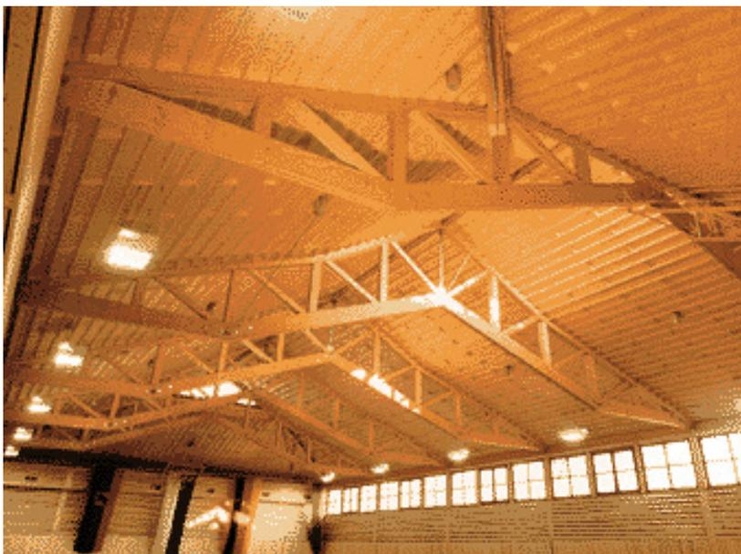
Fig. 6 Roof construction out of LVL-beams, Parkstein, Germany
