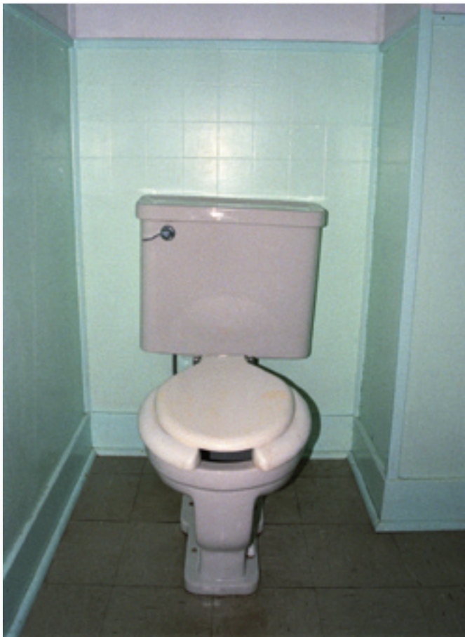
Figure 5—Temprrtile, a hardboard product embossed to resemble tile, was used as a water-resistant wainscot in the cook's bathroom at the Fenn Ranger Station.
