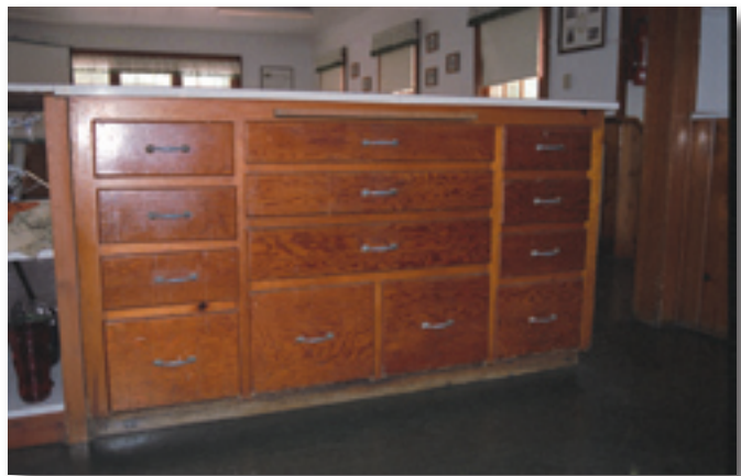
Figure 8—These plywood cabinets, constructed by the CCC in the cookhouse at the Fenn Ranger Station, are on the kitchen side of the serving counter. In this structure, cabinets visible only to the cook are plywood, while cabinets visible from the dining room are constructed of solid lumber.
