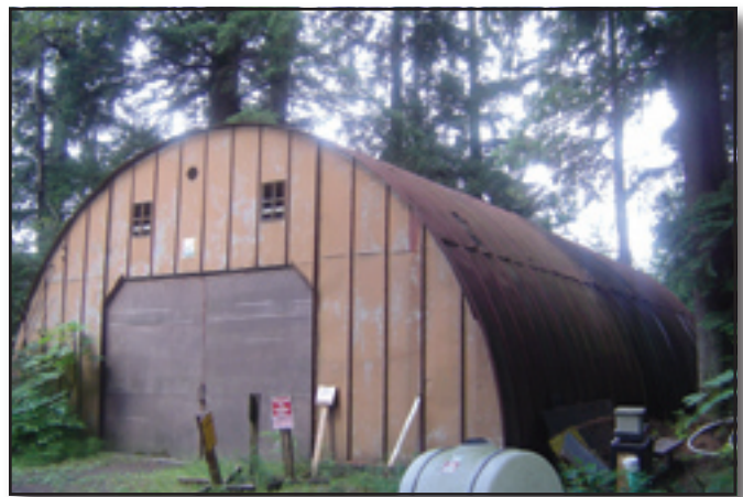
Figure 6—Masonite was often used to finish the interiors of the Quonset huts that the Forest Service acquired from the military after World War II. This Quonset hut is now used for storage at the Duck Creek Administrative Site (Juneau Ranger District, Tongass National Forest, Alaska Region).
