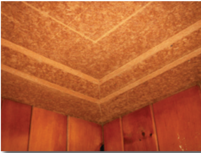
Figure 3—This fiberboard ceiling in the Butte Falls Ranger Station (Rogue River-Siskiyou National Forest, Pacific Northwest Region) has been carved into a decorative pattern. The ceiling is the natural brown color of the wood pulp from which it was manufactured.
