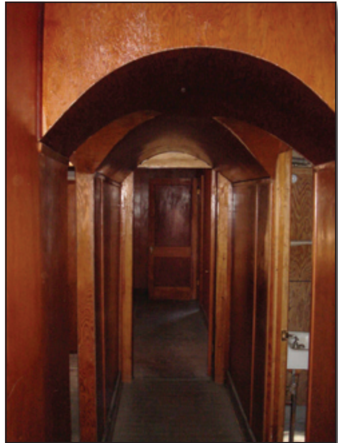
Figure 1—Varnished plywood covers the walls and ceiling of the Rabideau infirmary, which was built in 1935.
