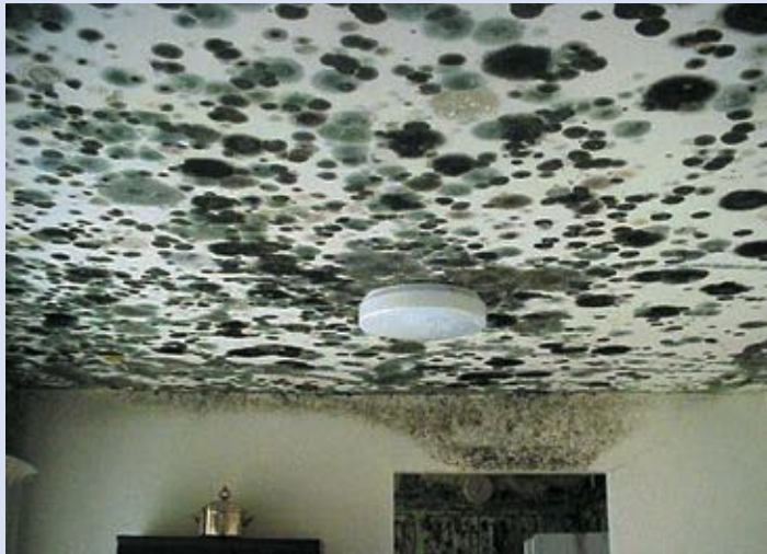
Photo 2: Extensive mold contamination of ceiling and walls
