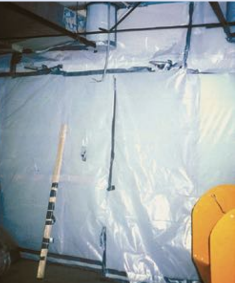
Photo 8: Full containment on large job
