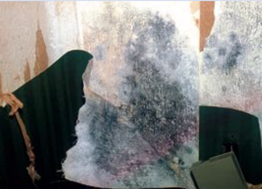
Photo 5: Mold growth behind wallpaper
