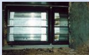
Photo 4C: Moldy air duct
