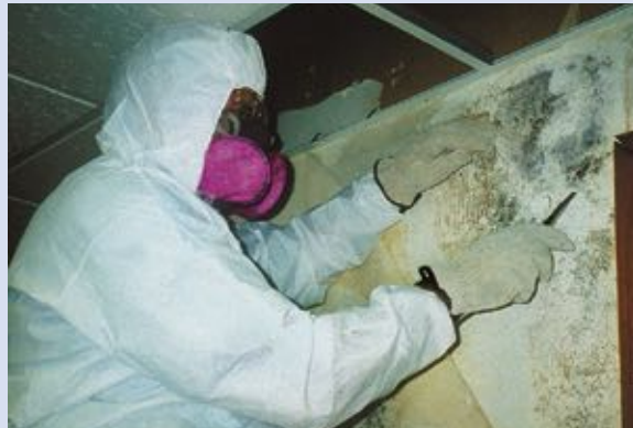
Photo 7: Remediation worker with limited PPE
