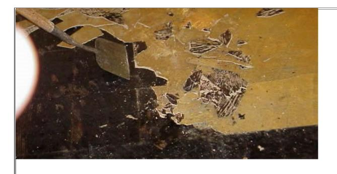
**Photo #8** - The floor tile in this picture may have been removed nonfriably and then placed in a lined fiber drum. The work crew used a hand tool to break up the floor tile in order to fit more into the drum. The floor tile has now become friable during the handling process. The floor tile needs to remain nonfriable from removal until it is disposed of.
