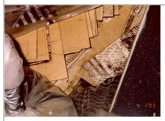
**Photos #3 & #4** - The asbestos-containing floor tile in these photos was removed with dry ice and an ice chipper. Too much breakage is occurring to the floor tile. MDH recommends reviewing and/or modifying work practices to reduce breakage.
