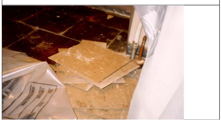
**Photo #2** - This asbestos-containing floor tile was removed with an ice chipper. The tile remained in whole pieces with little breakage.
