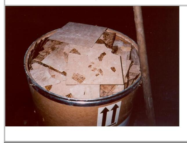
Photo #9 - The floor tile in this picture may have been removed nonfriably. Even though the floor
