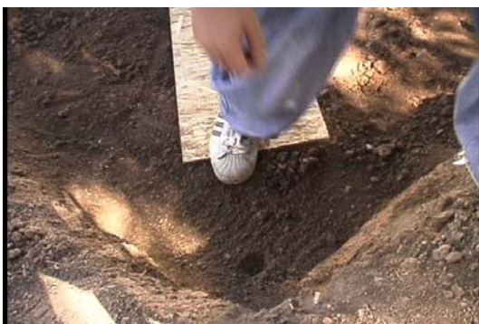
Figure 13. Trench bottom should be protected from extensive foot traffic using boards or planks.
