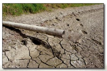
A horizontal pipe can't be used to its fullest potential until the pond level is too high. Unlike a vertical pipe, this type seldom will build a suction.
