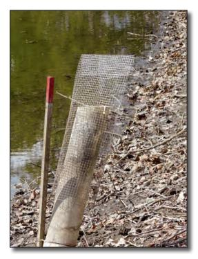
A vertical stand pipe or overflow like the above picture is the best and most effective. When the water level reaches the top of the pipe and runs over, the water will build up a suction or siphon effect and pull the water out. This is best on ponds that have a lot of watershed and can be quick to overflow.
