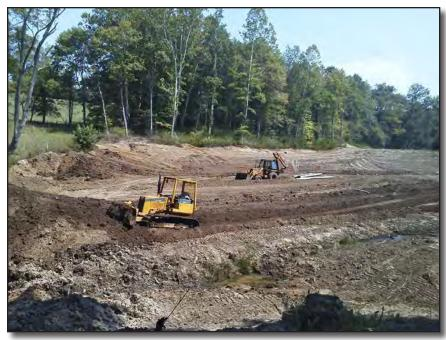
In this picture, I am in the process of pushing the dam up. If you have some rain fall while you are building the pond, it will help to always keep some slope in the bottom so if it does rain, the water will drain away. If the water can't drain away, you will have a muddy mess.
