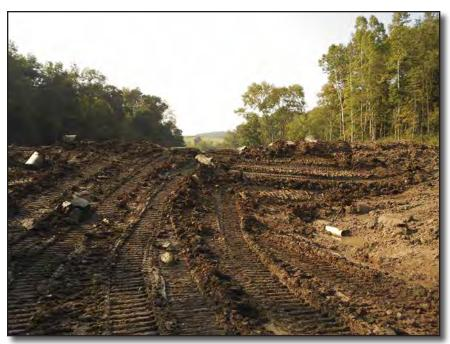
The picture on this page and the ones on the opposite page show the final stages of dirt back on the dam after the pipes have been installed.
