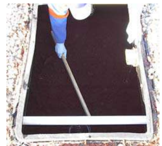
Leveling the Peat Moss
