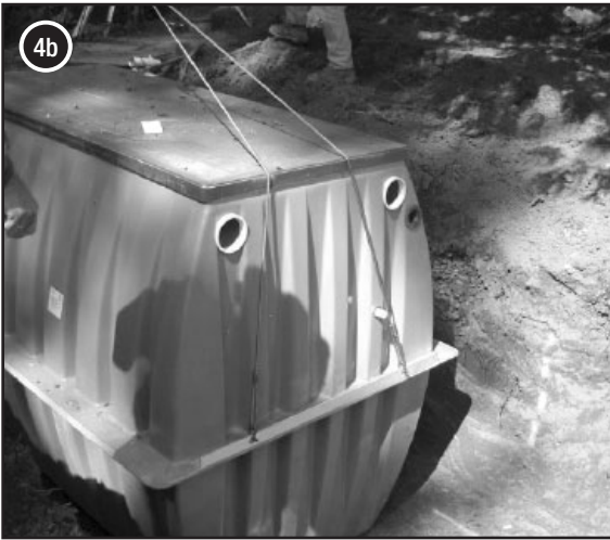
Lower the AX-RT unit into position.
