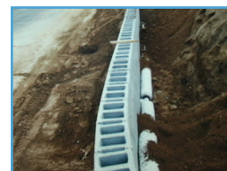
Retaining Wall Drain
