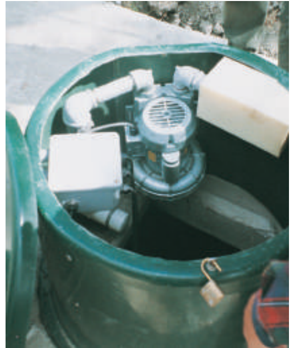
Aeration blower on an aerobic unit.
