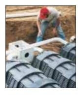
Gravel-less systems include SB2® pipe, Multi-pipe systems, GEO-flow pipe and HDPE leaching chambers. These are the most commonly used conduits in gravel-less systems.
