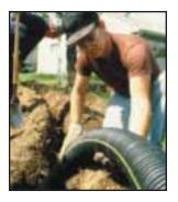
According the the EPA, the gravel in a conventional pipe and gravel system performs three basic functions: 1) its void spaces provide storage capacity for the effluent; 2) it protects the infiltrative surface area of the soil; 3) it supports the excavation. The gravel does not digest, treat or eliminate the effluent.
