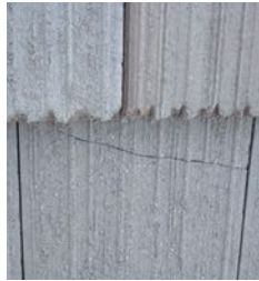
Roof tiles damaged by foot traffic or other types of damage should be replaced.
