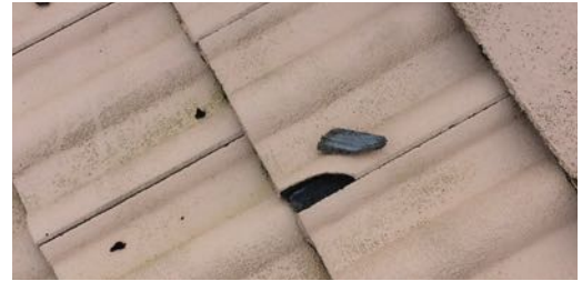
Small corner chips less than approximately 3" may be repaired by gluing the broken area in place.
