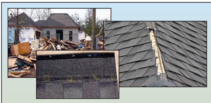
Figure 8-7. Loss of asphalt shingle roofing along hip. Best Practices approaches contained in Technical Fact Sheet No. 20 help prevent this mode of failure. (Source: FEMA 489)
