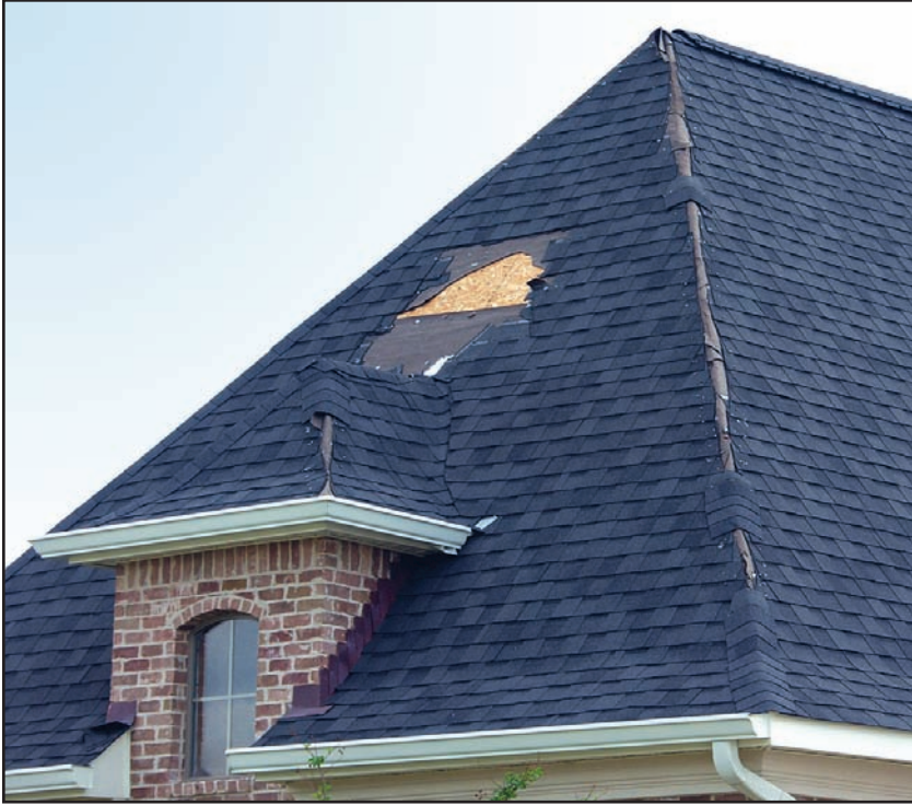
Figure 8-1. Instance where wind pressures exceeded the strength of the asphalt roofing. (Source: FEMA 549)
