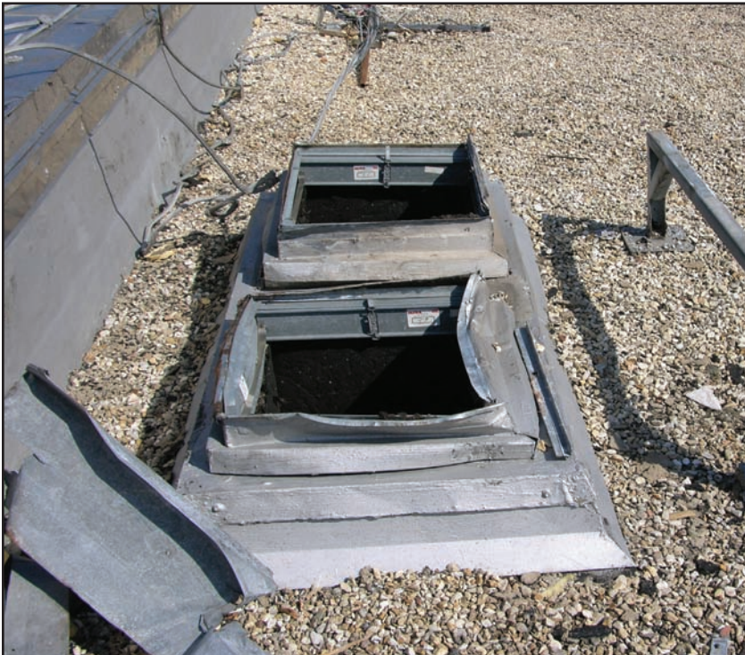
Figure 8-2. GULFPORT, MISSISSIPPI: Winds dislodged roof mounted equipment and created large openings in the roof system. (Source: FEMA 549)
