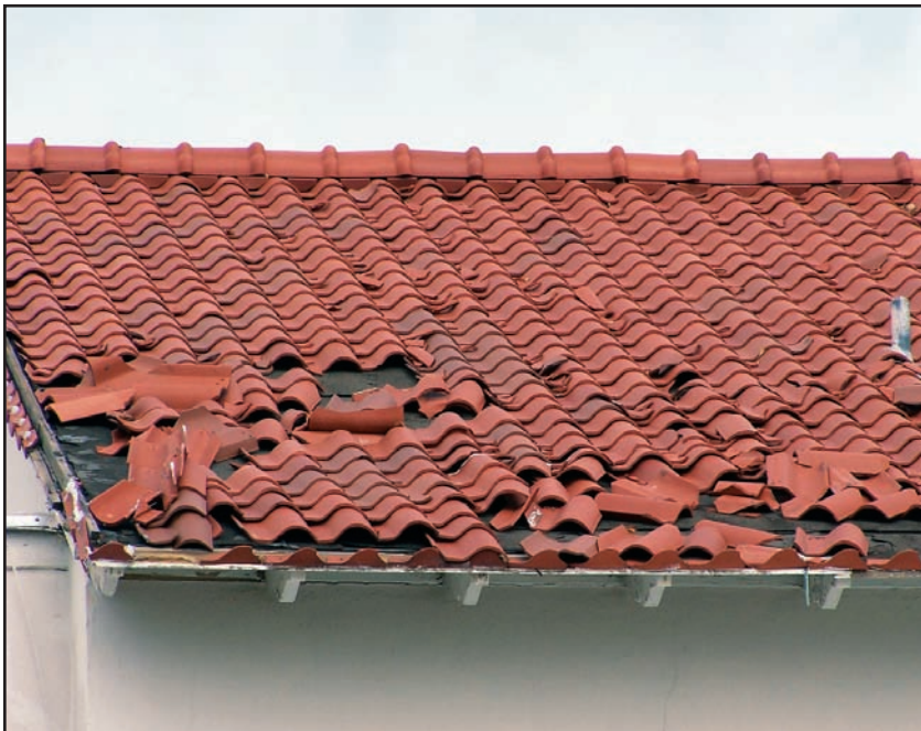
Figure 8-8. Clay tile roof failure. The tiles were dislodged due to inadequate anchorage. (Source: FEMA 549)
