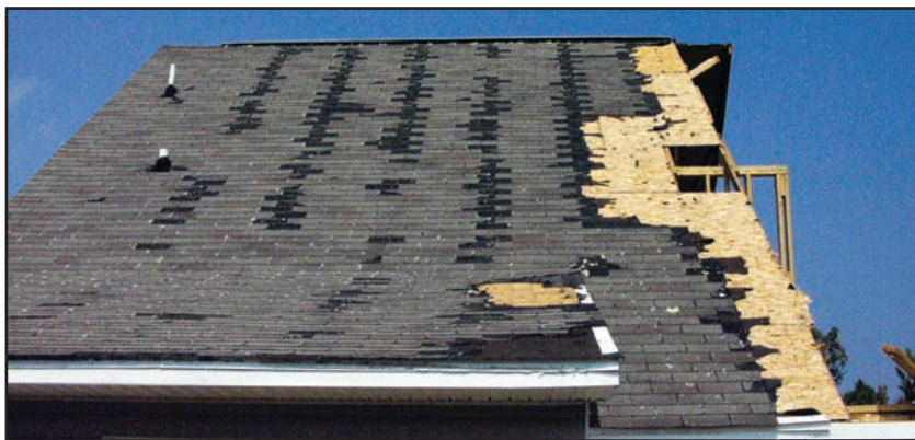
Figure 8-6. Roof failures that resulted from asphalt shingles being installed in a raking fashion. (Source: FEMA 489)
