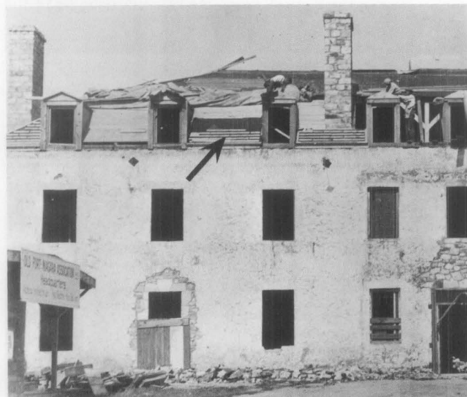
9. This 1927 view of the reshingling of the French Castle at Old Fort Niagara, N.Y., shows the wooden sleepers being laid (see arrow) over solid sheathing in order to raise the shingles up slightly to allow under-shingle ventilation. Note that the horizontal strips are not continuous to allow airflow and trapped moisture to drain away. This cedar roof has lasted for over 60 years in a harsh moist environment. Photo: Old Fort Niagara, Assoc. Inc.
