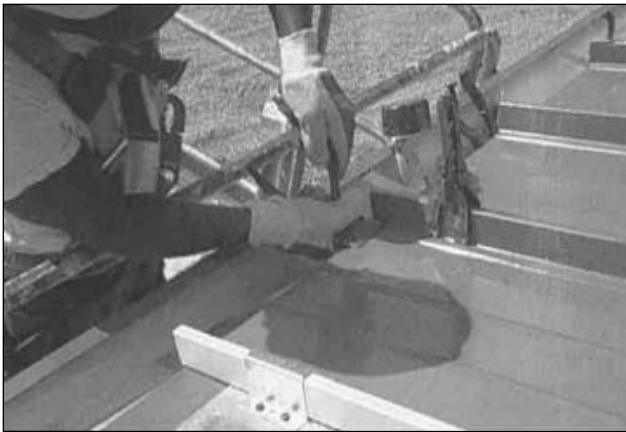
Figure 16-28 Spacer Tools Help Hold Panel Module
