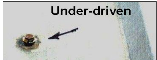
Figure 10-78 Under-Driven Fasteners Will Leak and Corrode
