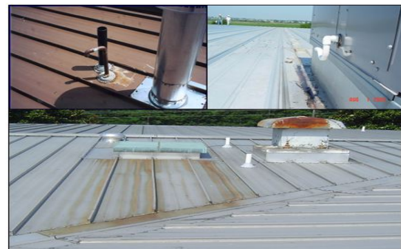
Figure 10-46 Staining and Corrosion from Copper Runoff
