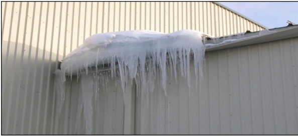
Figure 7-8 Possible Snow and Ice Effects Require Special Attention During Installation
