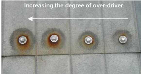
Figure 10-79 Over-Driven Fasteners
