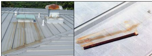
Figure 10-41 Corrosion Damage to a Metal Roof
