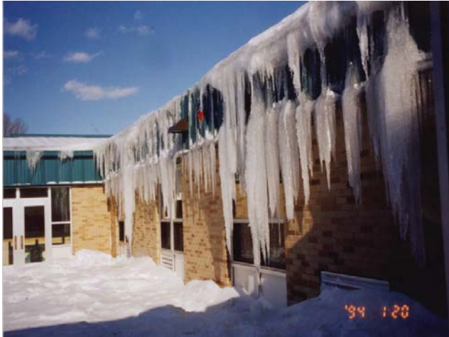
Figure 10-22 Undesirable Ice, Icicles, and Ice Dams
