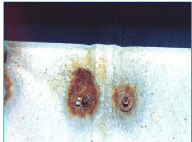
Figure 10-48 Incorrect Fastener Material
