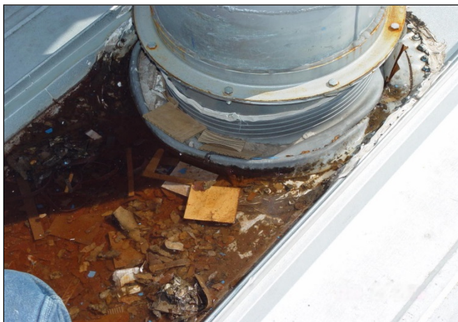
Figure 10-67 Improperly Installed Pipe Blocking Water Flow
