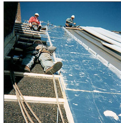
Figure 10-13 Installation of Rigid Polyiso Insulation
