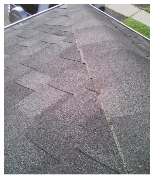
Combined with the apparent lack of chalk lines, this resulted in a messy-looking job. Using one of IKO's pretrimmed ridge cap products could have greatly improved this installation.
