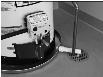
Figure 23 - Metal drain pan piped to drain.
