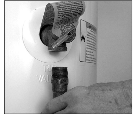
Figure 21 - Removing the T&P Relief Valve discharge pipe.
