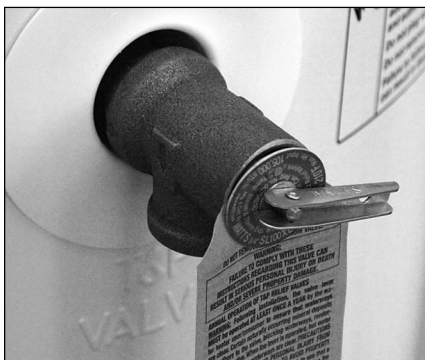
Figure 25 - Temperature and Pressure Relief Valve
