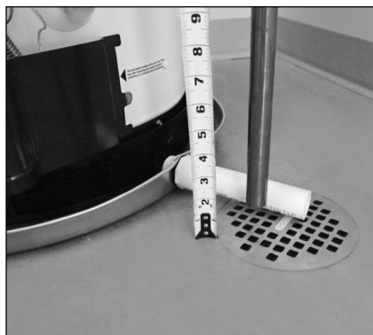
Figure 26 - Temperature and Pressure Relief Valve Pipe
