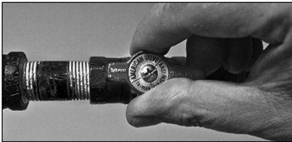
Figure 32 - Gas valve in "on" position
