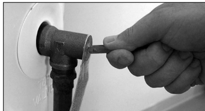
Figure 45 - T&P Relief Valve.
