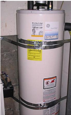
**Prevent gas leaks and water damage during an earthquake by properly securing your water heater as outlined in this bulletin.**
