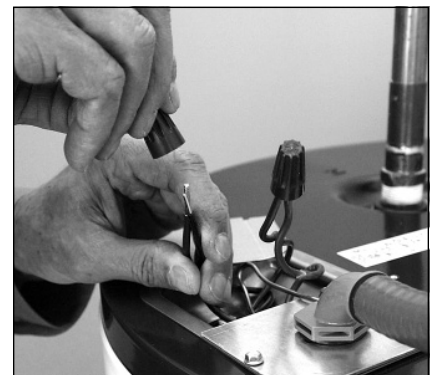
Figure 19 - Connecting the electrical wires.
