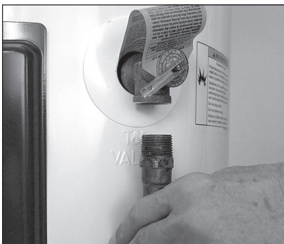
Removing the T&P Relief Valve discharge pipe.
