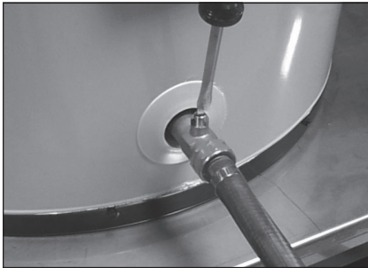
Draining the old water heater.
