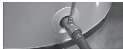
Figure 38 - Drain Valve
