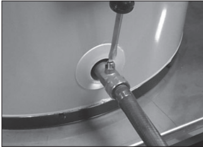
Figure 10 - Draining the old water heater.
