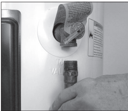
Figure 11 - Removing the T&P Relief Valve discharge pipe.
