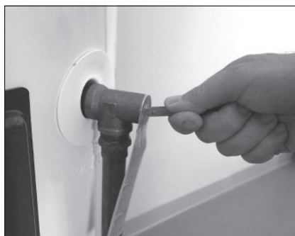
Figure 41 - T&P Relief Valve
