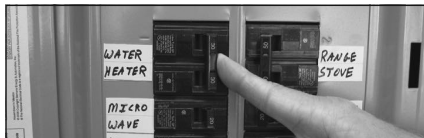
Figure 24 - Circuit Breaker
