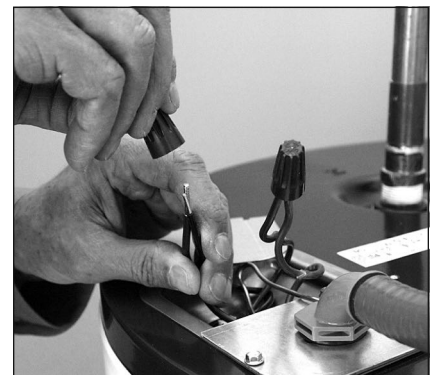
Figure 19 - Connecting the electrical wires.
