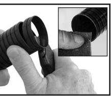
Cut the tube at the groove using a sharp utility knife to ensure a square, flat cut. Clean burrs from the cut end with emery paper.
