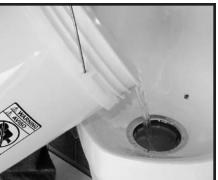
Pour 5 gallons of water as rapidly as possible into housing to ensure good flow and no leaks or standing water.
