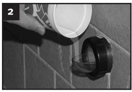
Clean face of existing wall flange then install the 2" compression nut with the clear inspection disc. Slowly pour water into the drain.
