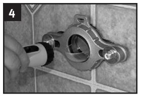
Use a flashlight to check pitch/slope. There should be no water present in the inspection disc or nipple. Remove flange after inspection.
