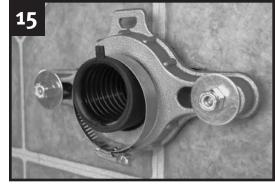
Install the gear clamp with the screw head at the bottom, but do not tighten.
