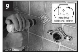
Drill two more holes for the hanger bracket, install screws, and tighten. Also drill holes for the lower anchor screws and insert plastic anchors.
