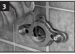
Clean face of existing wall flange then install the brass flange with the clear inspection disc. Slowly pour water into
