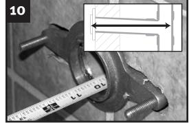
Determine the drain nipple depth by measuring the distance between the back of the sanitary tee (or elbow) to the front edge of the brass flange.
