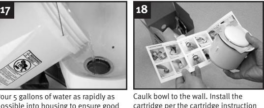
Pour 5 gallons of water as rapidly as possible into housing to ensure good flow and no leaks or standing water.
