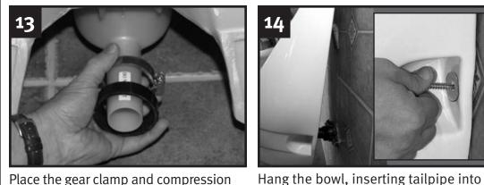
Place the gear clamp and compression nut onto the housing tailpipe. Apply lubricant to the tailpipe.
