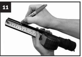
Find the drain nipple depth on the cutting chart (left) and mark the specified trim length on the insert tube at the nearest 1/4" groove.
