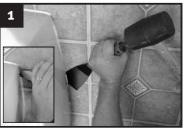
Use utility knife to cut caulk, then use a putty knife and mallet to remove the bowl. Remove hanger brackets, scrape off caulk, and clean the wall.
