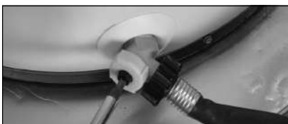
Figure 42 - Draining the water heater.
