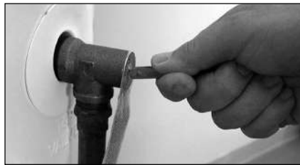
Figure 45 - T&P Relief Valve.
