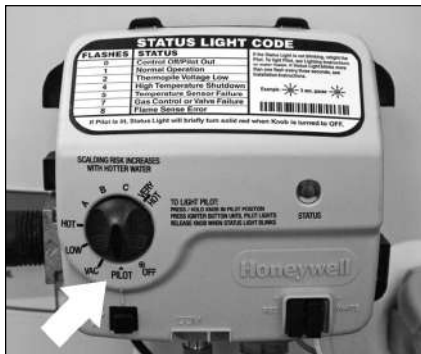
Figure 48 - Gas control/valve.
