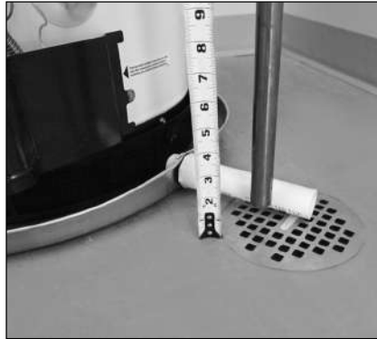
Figure 26 - Temperature and Pressure Relief Valve Pipe
