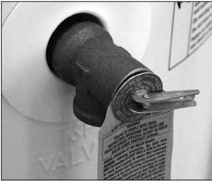
Figure 25 - Temperature and Pressure Relief Valve
