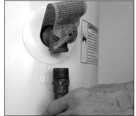
Figure 21 - Removing the T&P Relief Valve discharge pipe.
