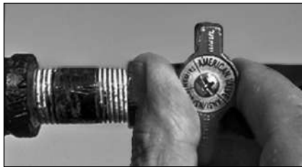
Figure 50 - Gas valve in “off” position.
