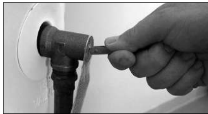
Figure 45 - T&P Relief Valve.
