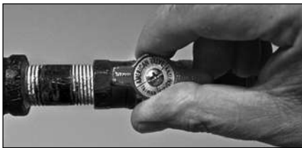
Figure 32 - Gas valve in "on" position
