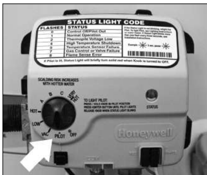
Figure 48 - Gas control/valve.
