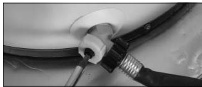
Figure 42 - Draining the water heater.
