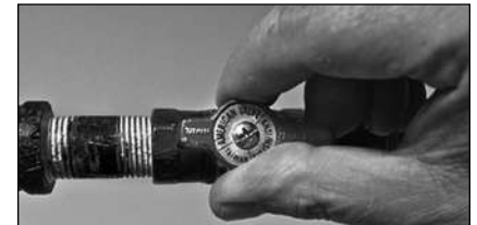
Figure 58 - Gas valve in “on” position.
