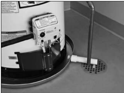
Figure 23 - Metal drain pan piped to drain.
