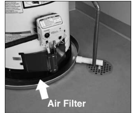
Figure 24 - Filter attached to water heater.
