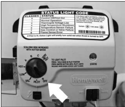
Figure 40 - Turn gas control/temperature knob OFF.
