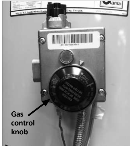
Figure 17 - Turn gas control/temperature knob OFF.
