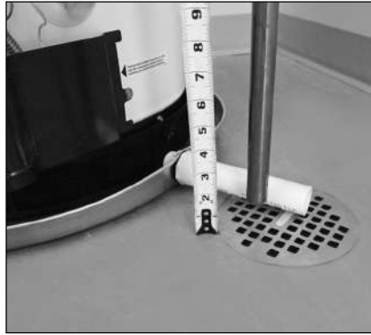
Figure 26 - Temperature and Pressure Relief Valve Pipe
