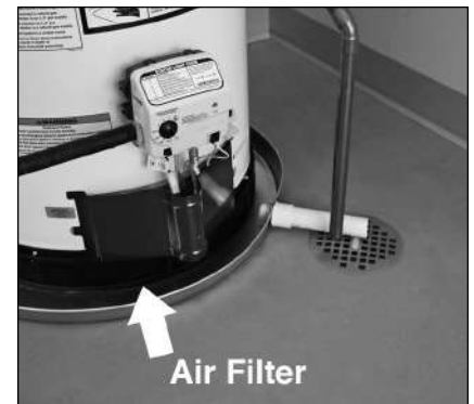
Figure 24 - Filter attached to water heater.
