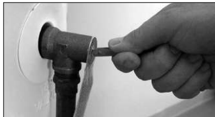
Figure 45 - T&P Relief Valve.
