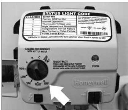
Figure 40 - Turn gas control/temperature knob OFF.
