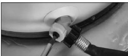
Figure 42 - Draining the water heater.
