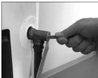
Figure 38 - T&P Relief Valve
