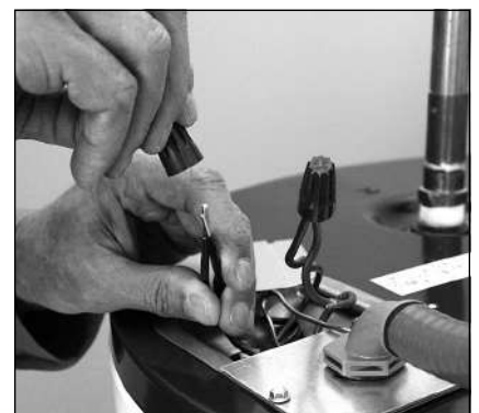
Figure 19 - Connecting the electrical wires.
