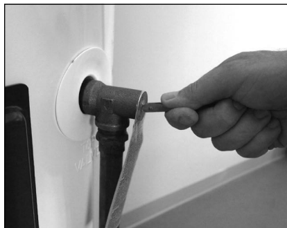
Figure 38 - T&P Relief Valve
