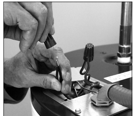
Figure 19 - Connecting the electrical wires.
