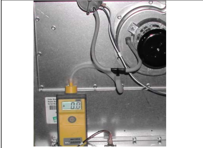
FIGURE 9: Single Port Pressure Switch
