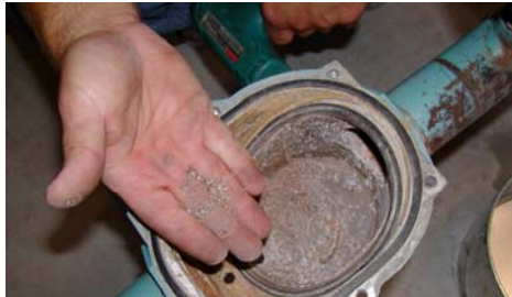
Dirt and Scale in a Fuel Gas Safety Shutoff Valve
