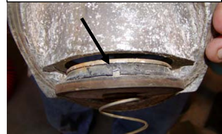
Gashed Rubber Seat in a Diaphragm type Safety Shutoff Valve.
